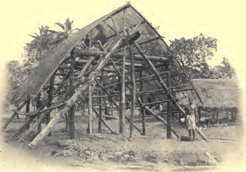
BEGINNING TO BUILD A SAMOAN HOUSE.
